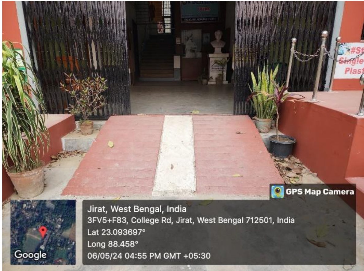
Ramp at the entrance of the main building
