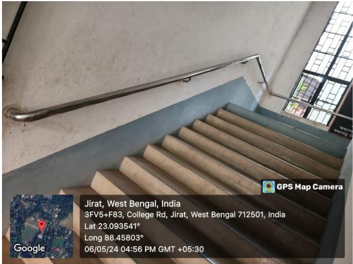
Railing in staircases
