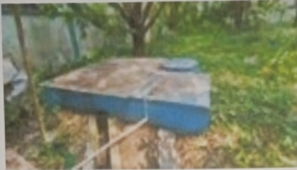
The Rainwater harvesting facility in the College ground
