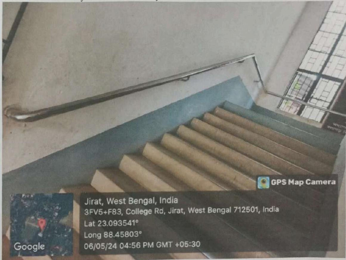
Railing in staircases
