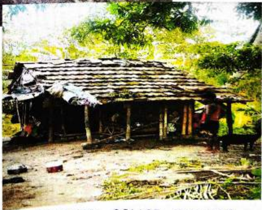
TEMPORARY RELIEF SHELTER OF EROSION EFFECTED PEOPLE
