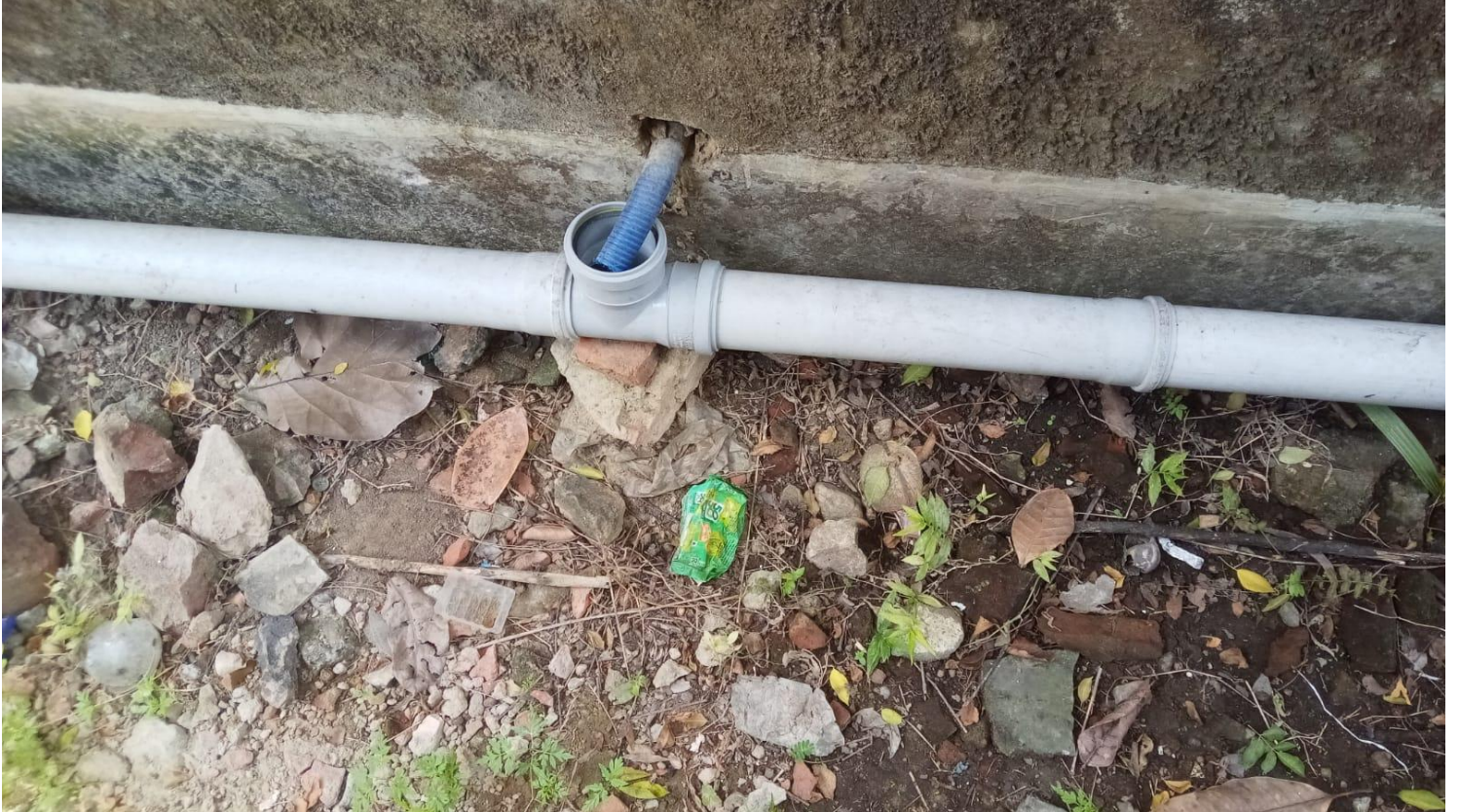
Pipe Line Connection for Rain Water Harvesting in College Campus
