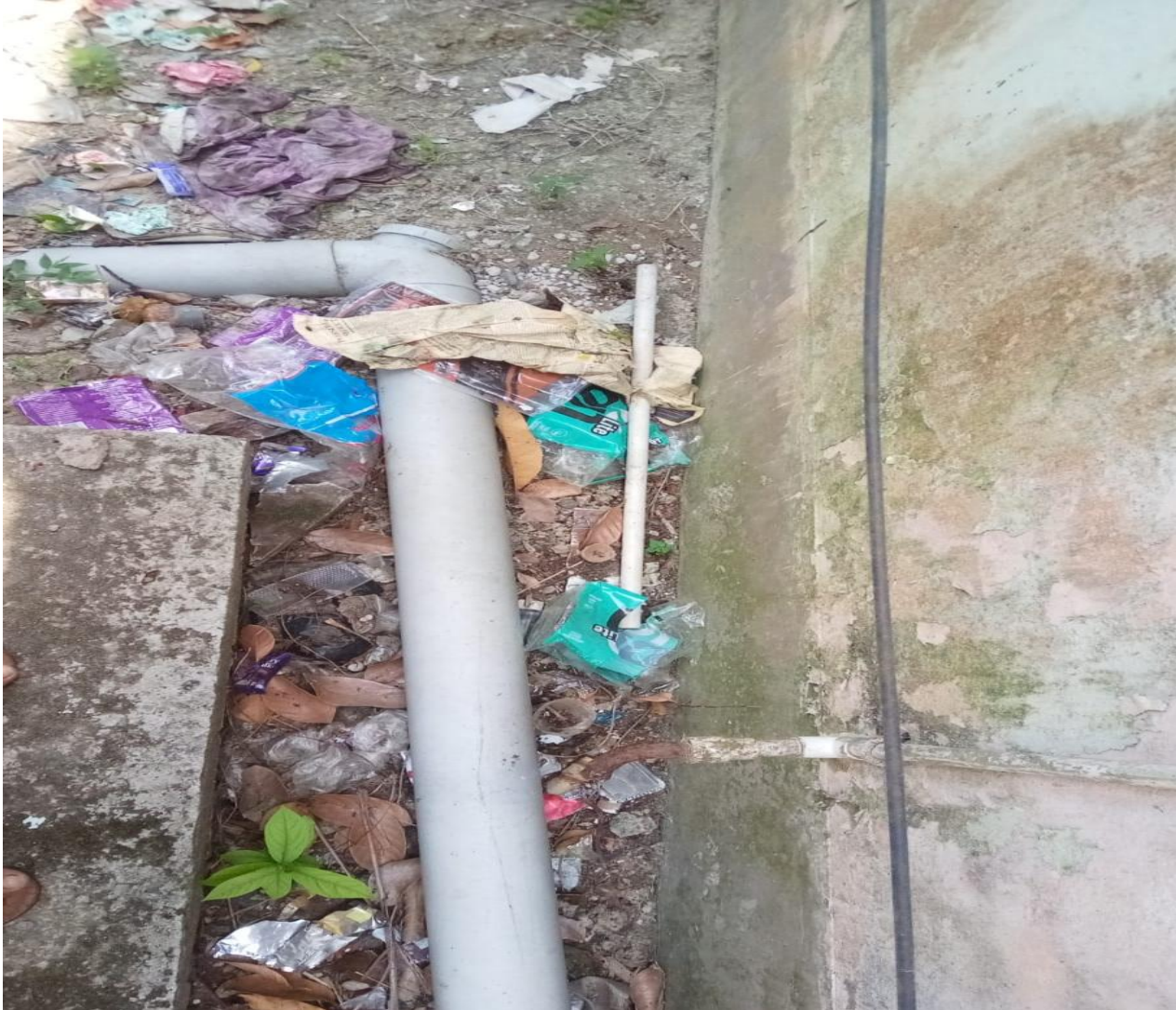
Pipe Line Connection for Rain Water Harvesting in College Campus
